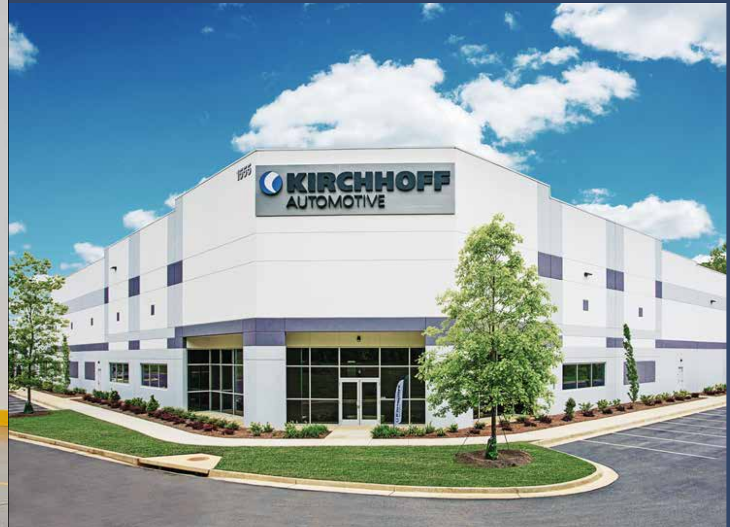
The newly opened KIRCHHOFF Automotive plant in Atlanta, North America.
