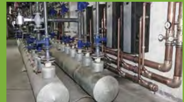
Fresh water modules for drinking water heating using the instantaneous water heater principle with cascade control.
