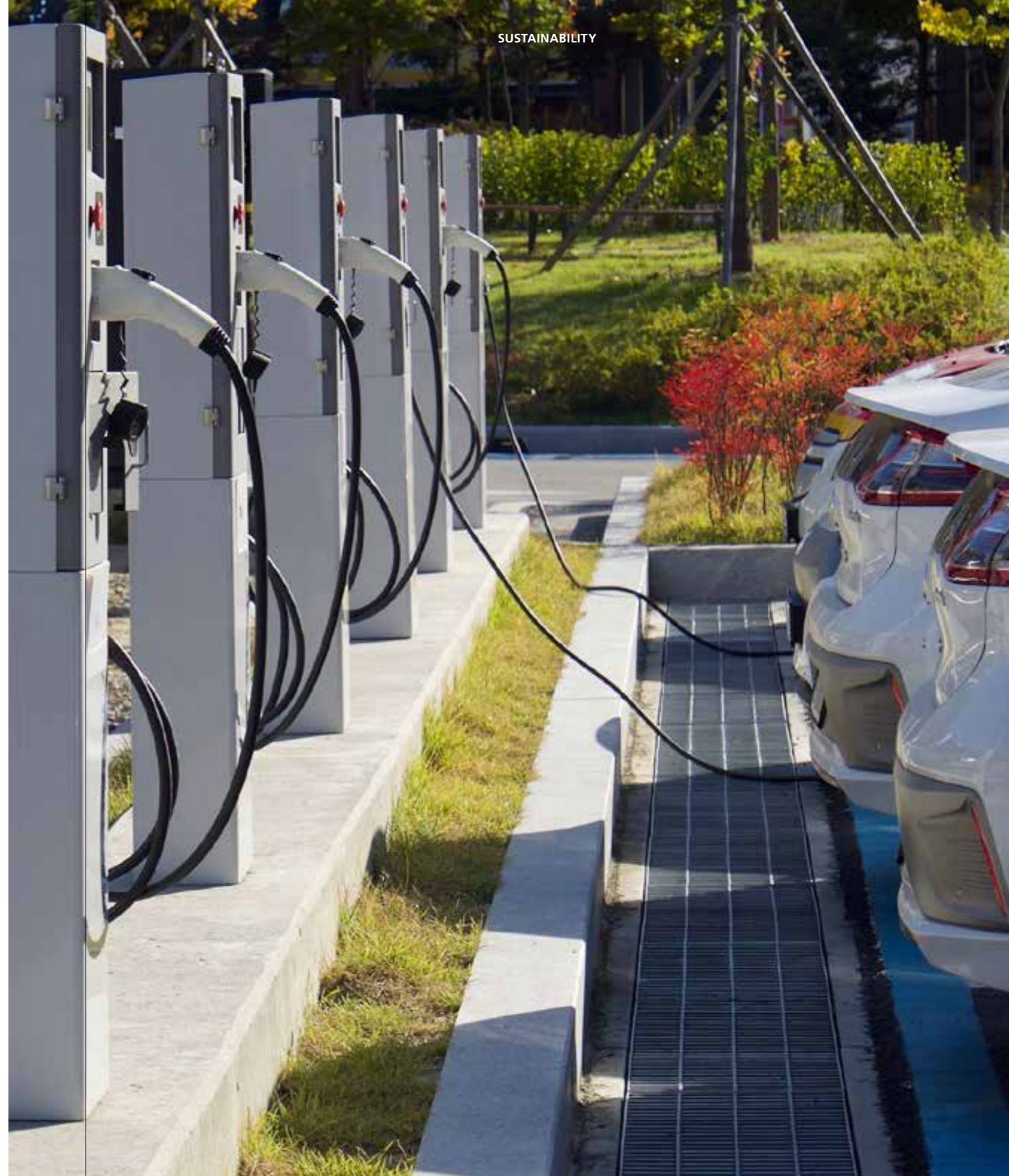
The charging stations are often difficult to reach for wheelchair users with vehicles standing close together. Photo Credit: EMG (European Mobility Group) https://www.mobilitygroup.eu/news/europe-ready-electric-revolution
