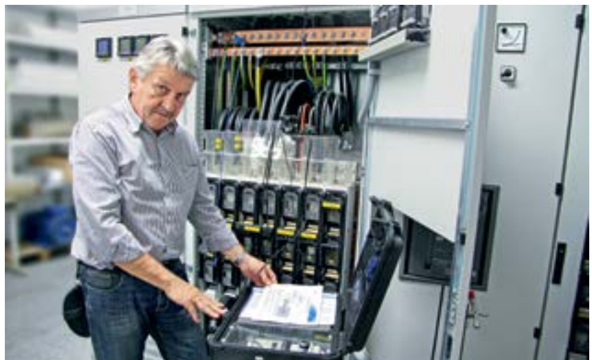
Dieter Hoffmann, energy officer for Iserlohn, checks the energy consumption with a special portable measuring set.
