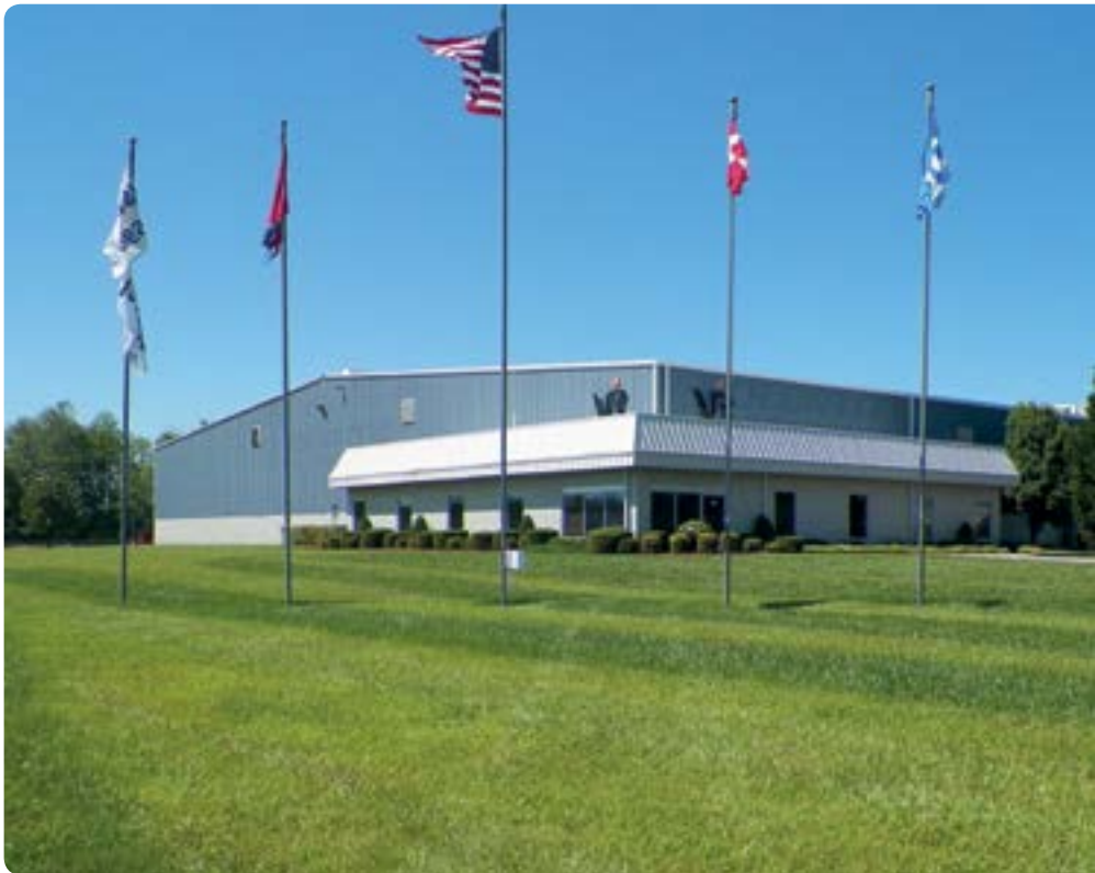
The Manchester plant before the expansion.
